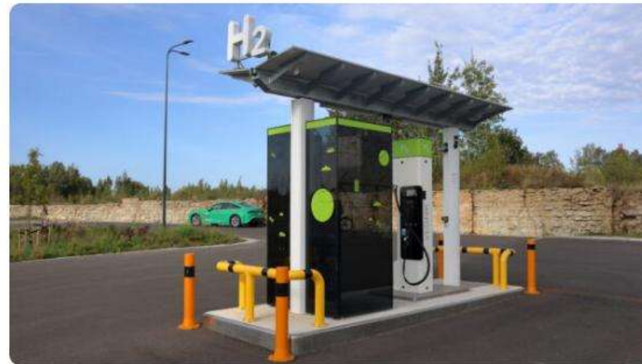
Hydrogen Refueling Station in Tallinn
